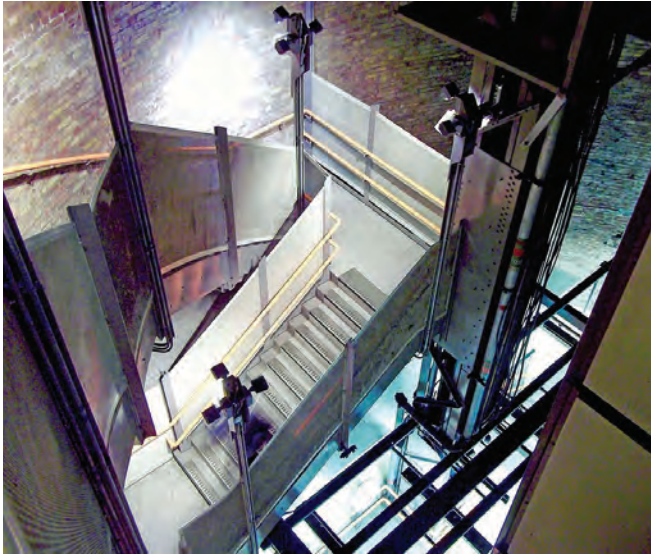
The shaft is still in use for platform access
